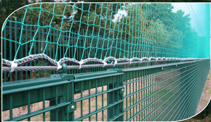
Detail of Ballstop fixing to top of Pro-Sport Fencing System
